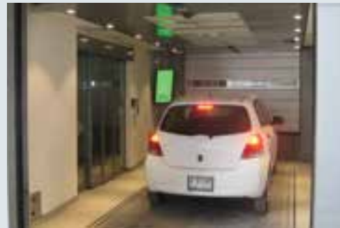
Entrance transfer area - car is lifted and transported to parking space
