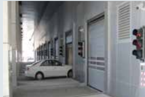
Cars enter through openings with high speed roll-up doors - traffic lights signal when it's safe to enter
