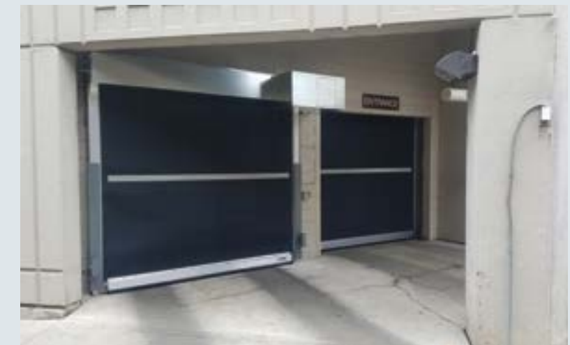
Rugged SBR rubber panel provides outstanding performance in abusive environments
