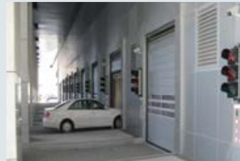
Cars enter through openings with high speed roll-up doors - traffic lights signal when it's safe to enter
