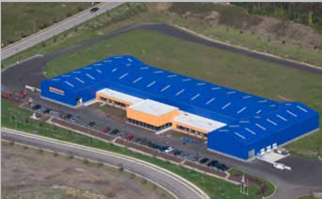
Hörmann Flexon LLC, Burgettstown, PA Headquarters and Manufacturing Plant
