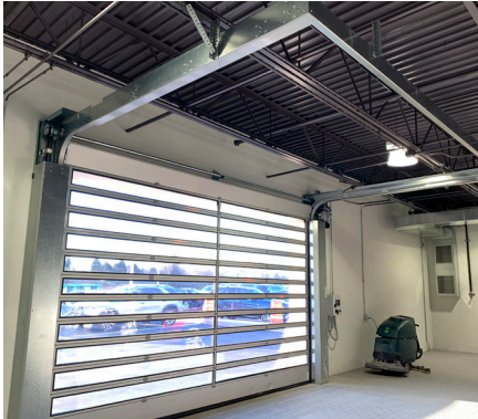
Speed-Guardian™ Low Headroom, high-speed doors provide excellent capability in low-clearance areas.
